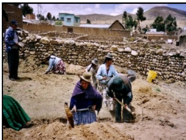
Community members may lay over two miles of piping to bring water to every house.
